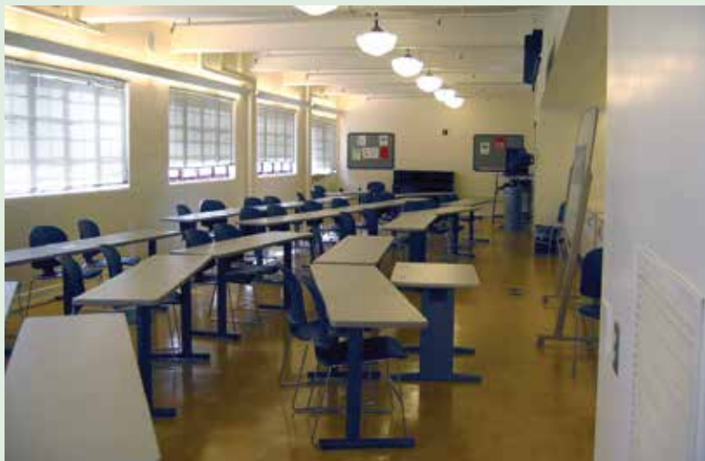
TOP Renovations in the Bell Tower begin. ABOVE Classrooms in the Bell Tower are narrow.
